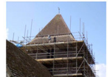
12 Tower roof retiling in progress [4.9.19]
